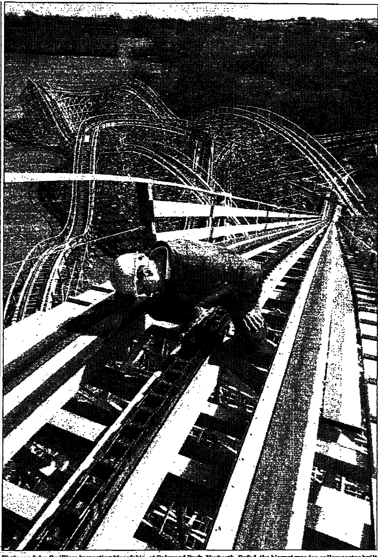
Engineer John Gwilliam inspecting Megafolia, at Oakwood Park, Narberth, Dyfed, the biggest wooden roller coaster built in Europe in 50 years. It opened on Saturday after tests using a computerised dummy passenger. PHOTOGRAPH: JEFF MORGAN
